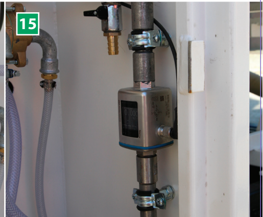
15 Flow measurement chemistry (option) Electromagnetic flow measurement, 1/2" in stainless steel, max. 16 bar, temperature -10 to +70 °C, minimum conductivity 20 µS / cm. The flow measurement guarantees a dosing accuracy to +/- 2 % (repeatedly +/- 0.2 %), according to EN 206-1.
