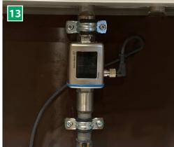
Flow measurement chemistry (optional) Electromagnetic flow measurement, ½" in stainless steel, max. 16 bar, temperature -10 to + 70 ° C, minimum conductivity 20 μS / cm. The flow measurement guarantees a dosing accuracy to +/- 1 % (repeatedly +/-0.2 %), according to EN 206-1.
